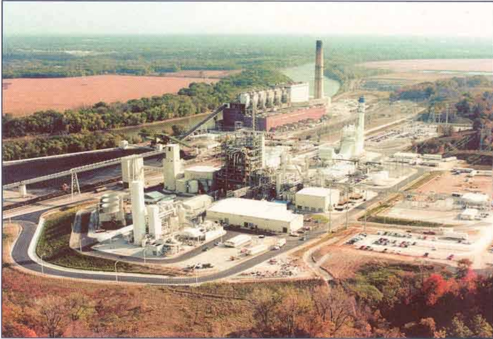
The Wabash River Coal Gasification Repowering Project
